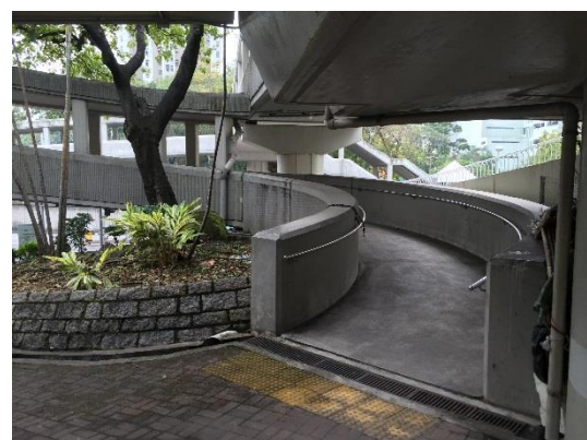
Figure 2.2 Footbridge in Tsuen Wan
