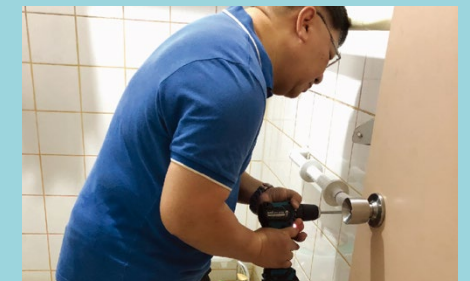
(Above and below) Volunteer technicians carrying out improvement work
